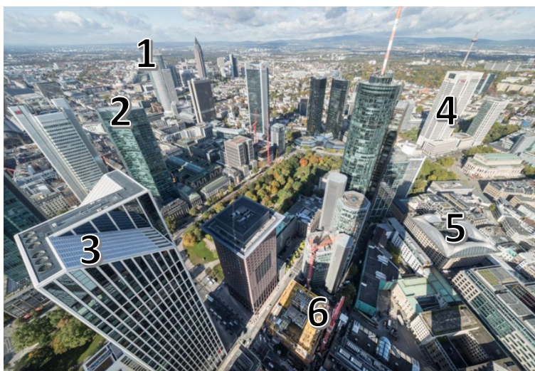
Figure 2. Skyscrapers No. 1 ... 5 referred to in Table 2 and construction site of skyscraper „Omniturm“ No. 6 (picture source [15])
